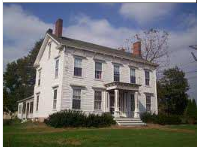
Hageman House, South Middlebush Road
